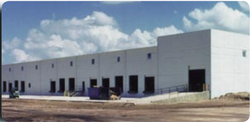
Nabisco facility construction underway
